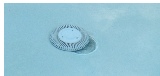
Figure 2: Drain cover that is loose.
