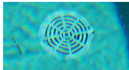
Figure 3: Non-approved drain cover.
