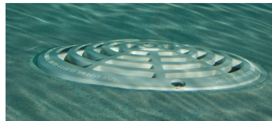
Figure 1: Approved drain cover, properly secured.
