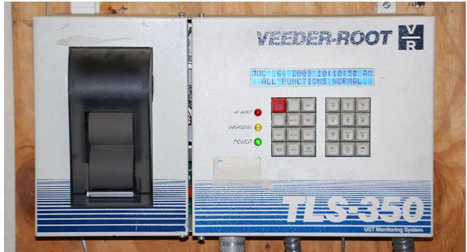
The difference between a monitoring system for a SWT and a DWT are no annular sensor and Continuous System Leak Detection (CSLD) for SWTs.
