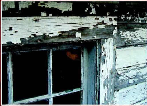
Deteriorated Lead Based Paint
