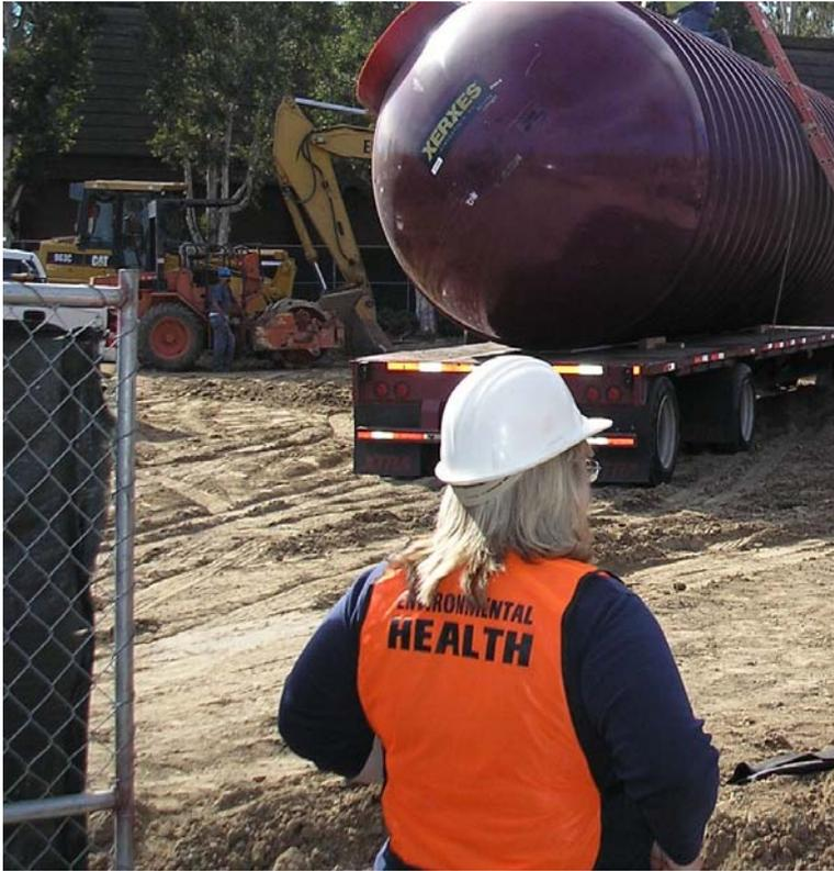
Depending on the upgrades to the underground storage tank (UST) system, a plan check submittal, inspection and fees to the County may be required. No matter what the upgrade is, a witnessed monitoring system certification is required to verify all monitoring parameters are met.
