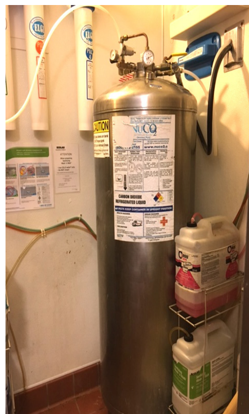
NuCO2 Bulk Liquid CO 2 cylinder, this is a 4000 CF (or 54 gallon) cylinder.
