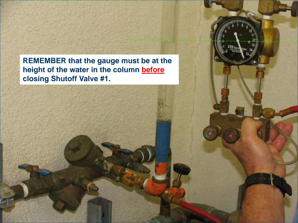
Making sure your gauge is at the highest point of water, open No. 3 test cock, record the gauge reading after it settles.
