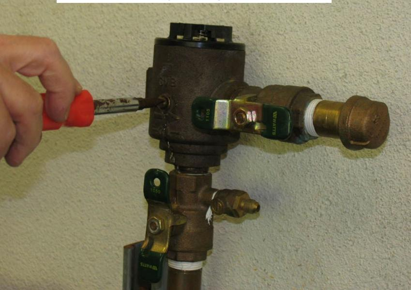
Attach the gauge to the bleed T and open the test cock. /
