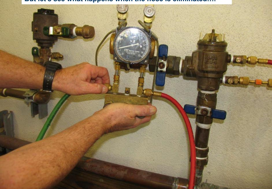
With the hose removed, the pressure drops to 0.0!
