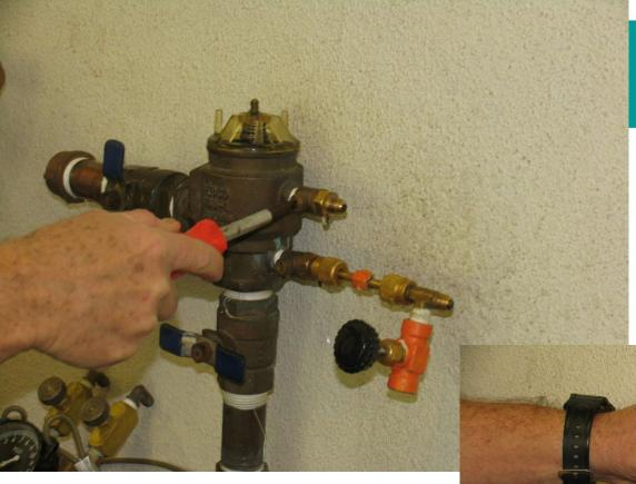
Close the No. 2 test cock and turn on Shutoff Valve #1 to pressurize the device.
